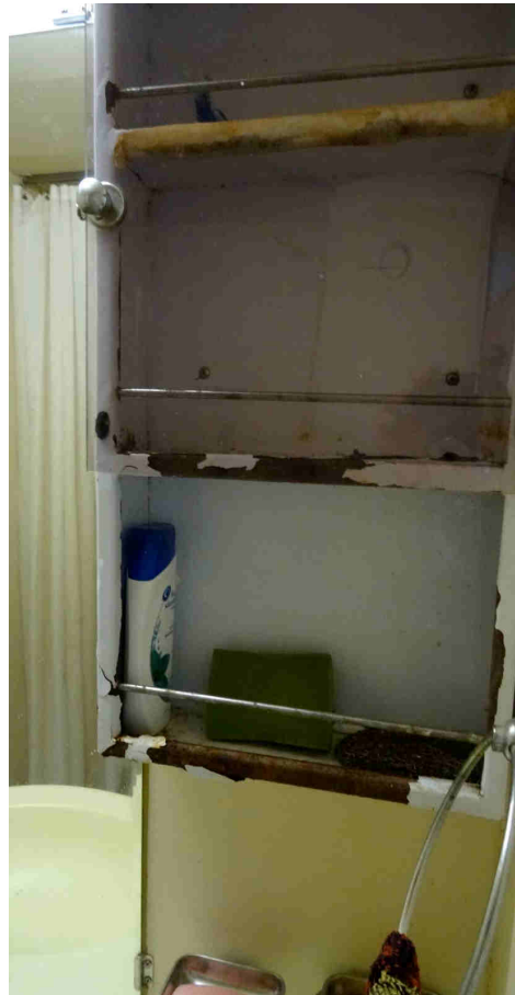
picture 17-19: in crew cabins all racks rusted and/or damaged; mould in all corners
