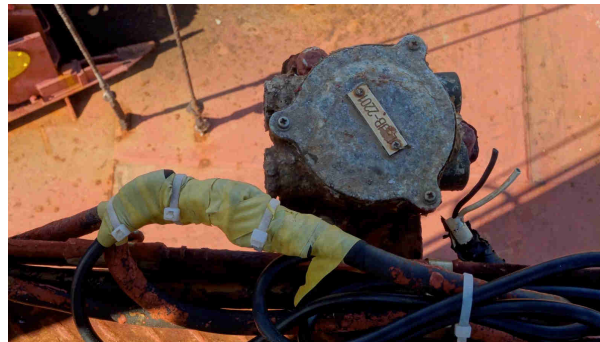
picture 8: self made connections.
