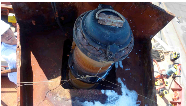
picture 2: second toplight, more wires necessary
